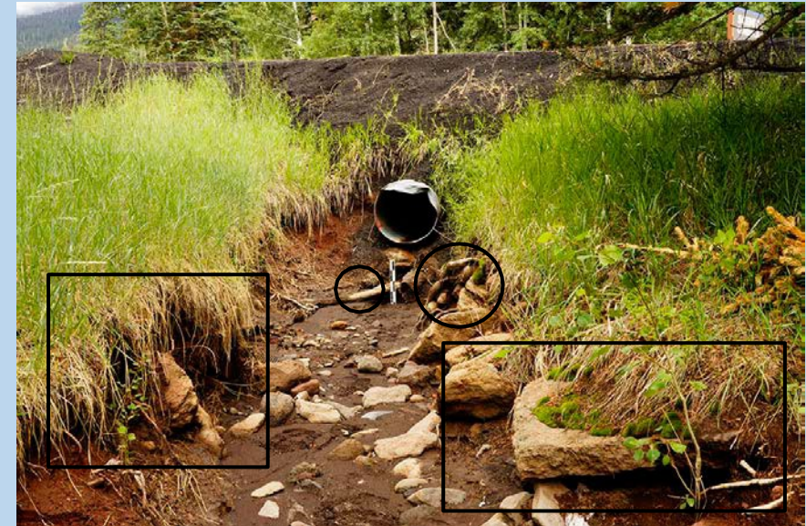
Upstream views of lower drainage system at and downstream of culvert. Upper left 9/20/2020 upper right 7/27/2021, scale 50 cm long with 10 cm (~4 inches) divisions. Common features are circled. Gully is deeper and substantially wider (rectangles).
