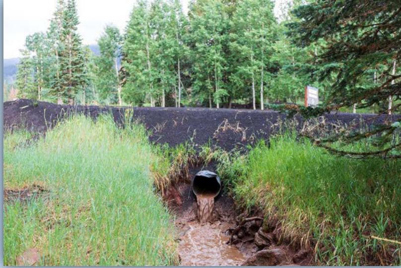
Drainage culvert flowing into previously eroded gully on Hart Prairie, July 18, 2021 around 4 pm. Culvert passes under Forest Road 516. Water quality samples were collected here just outside of Snow Bowl's permit area.
