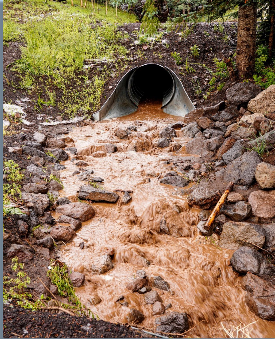
Left—Turbid, reddish brown runoff of August 14, 2022. The degree of turbidity is partly related to sediment concentration. Right—Continuation of the runoff as it flows in the open channel around the new parking lot and onto Hart Prairie.
